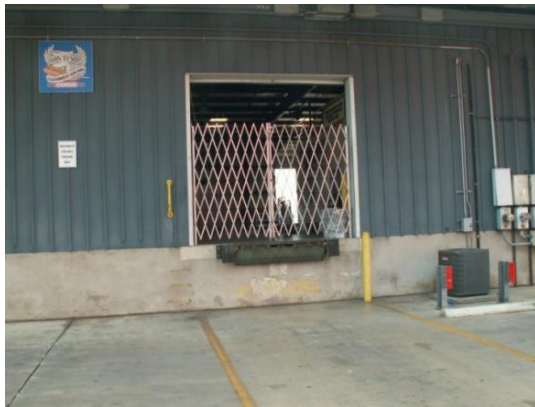
Figure 7-1. Scissor Gate on Public Side of Building
