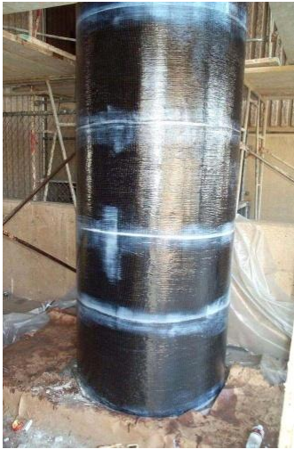
Figure B-11. Column Wrapping Procedure
