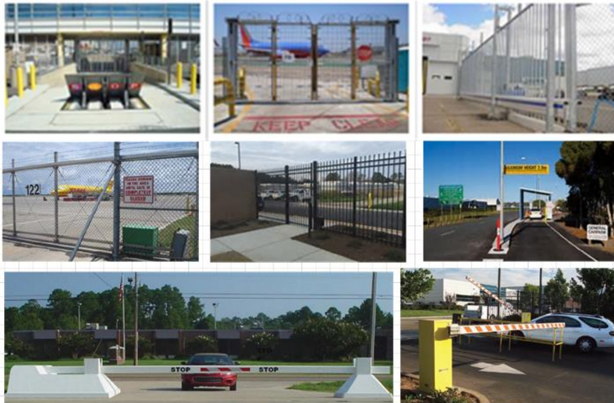
Figure 11-2. Examples of Airport Gate Installations
