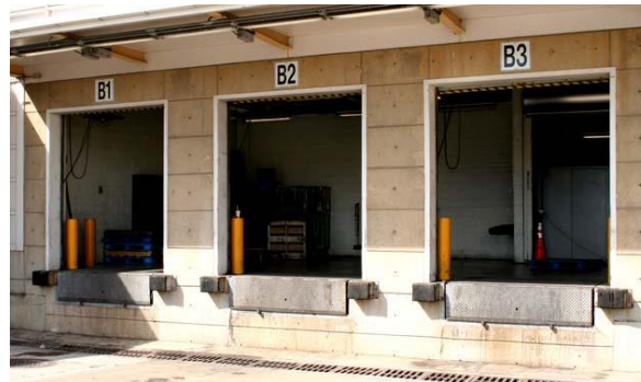
Figure B-6. Loading Dock
