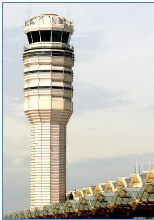
Figure B-8. ATC Tower
