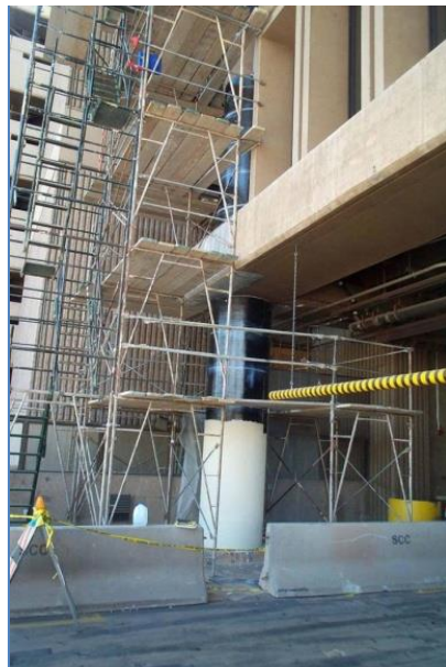
Figure B-4. Wrapping Process—Kevlar-Carbon Fiber Wrap
